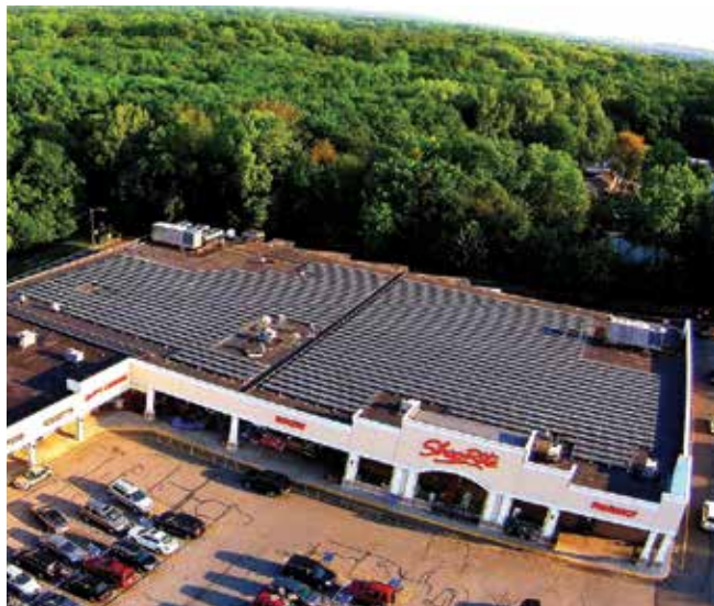
Emerson Shopping Plaza Emerson, New Jersey
