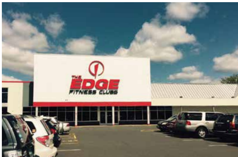
Dock Shopping Center Stratford, Connecticut
