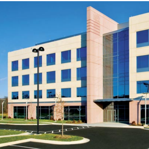
302, 304 and 306 Sentinel Drive at The National Business Park ( far left ) and 5825 University Research Court at M Square all achieved LEED Silver certification.
