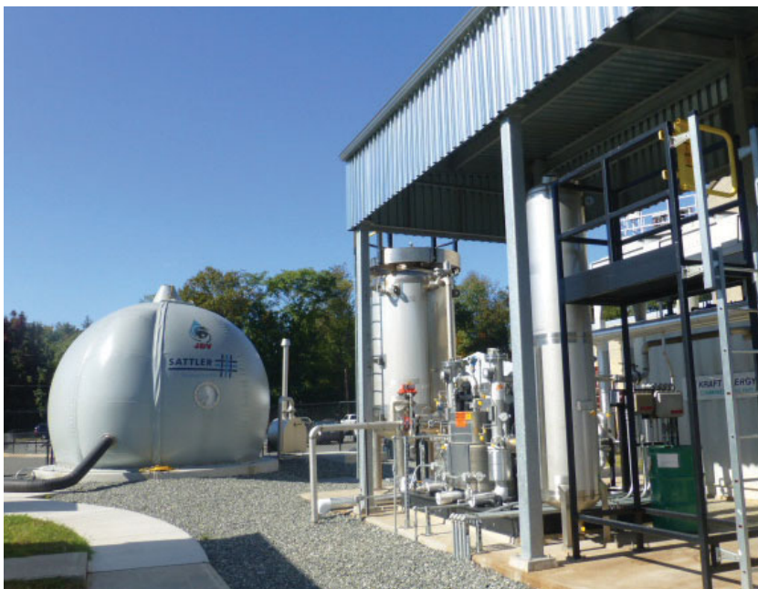
The biogas system at the Village of Ridgewood Water Pollution Control Facility became fully operational in 2013 and produces electricity from methane. The renewable energy project has resulted in utility costs savings and reduction in the Village's carbon footprint.
