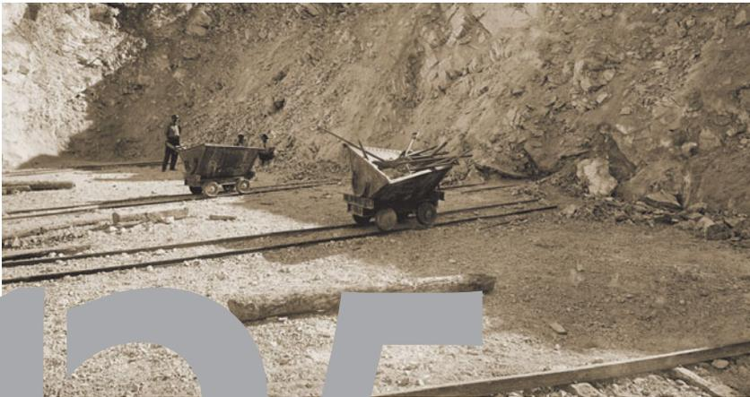
Miners take a short break at a small-scale open pit mine in 1918. Note the hand tools in the rocker dump cars: shovels for moving material, ballast forks for sifting rock.
