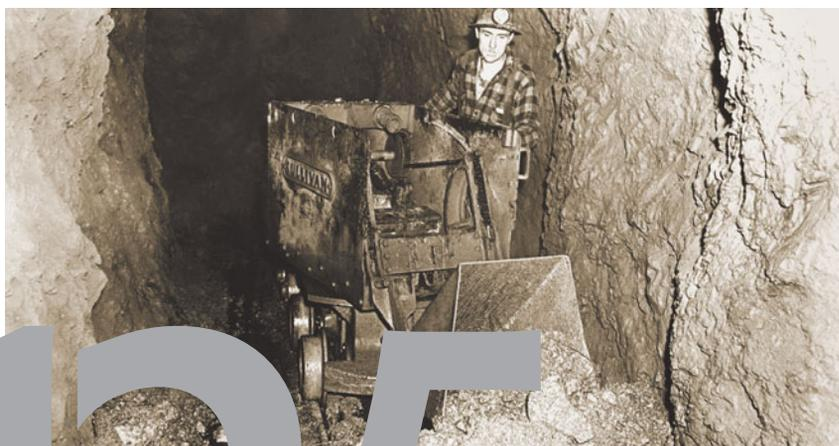
A miner operates a 4,200-pound mine-car loader deep underground in the Silver Valley. Introduced by Sullivan Machinery Co. in 1938, the portable, pneumatic HL-1 “mucker” was specially designed to load on sharp turns. Ca. 1950.
