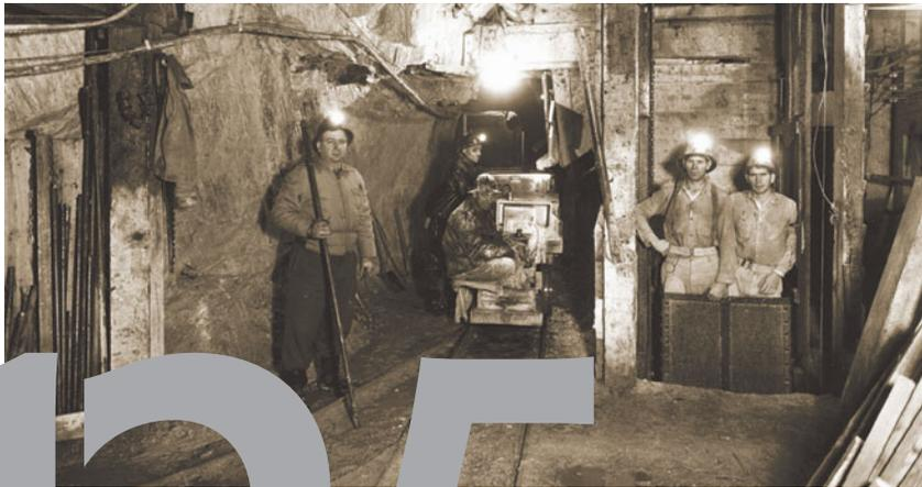
Workers underground at the Lucky Friday mine, 1945. The timber-framed skip in the #1 Shaft top station, at right, is just large enough to accommodate two miners. The current Silver Shaft can accommodate up to 17 miners.
