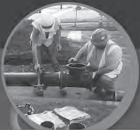
Water Main Replacement
