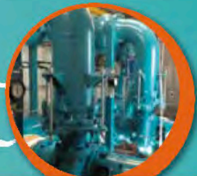
Booster Station Improvements
