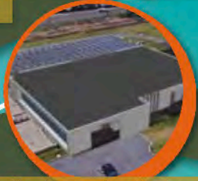
Water Treatment Plant Upgrades
