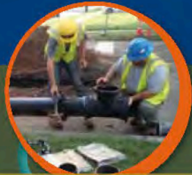
Water Main Replacement
