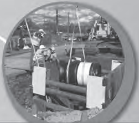
Secondary Transmission Main Construction
