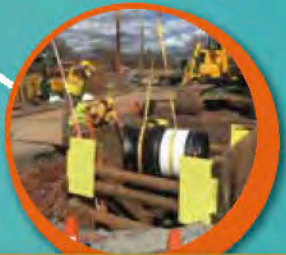
Secondary Transmission Main Construction
