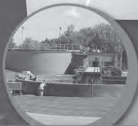
Wastewater Treatment Plant Contract Operations
