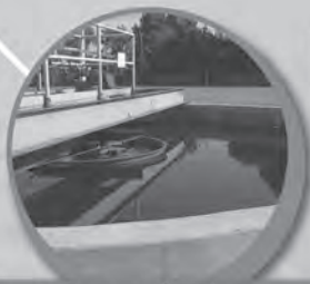
Wastewater Treatment Plant Improvements
