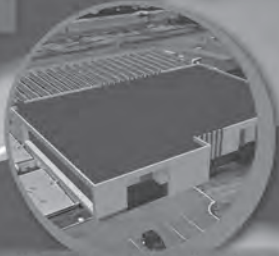
Water Treatment Plant Upgrades
