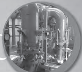
Booster Station Improvements
