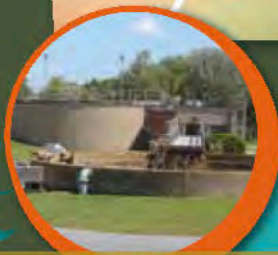
Wastewater Treatment Plant Contract Operations
